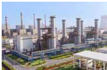
Bin Qasim Power Station II (573MW Combined Cycle). 3 x GE Frame 9E Gas Turbines & 1 Harbin Steam Turbine.
