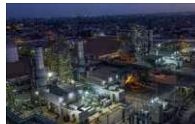
Korangi Combined Cycle Power Plant (248MW Combined Cycle). 4 x GE LM 6000 Gas Turbines & 2 x GE Steam Turbines
