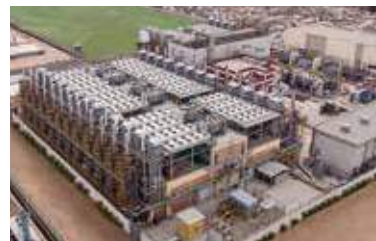
KGTPS-II (107MW Combined Cycle) 32 x GE JENBACHER Gas Engines & 1 x NG Allen Steam Turbine
