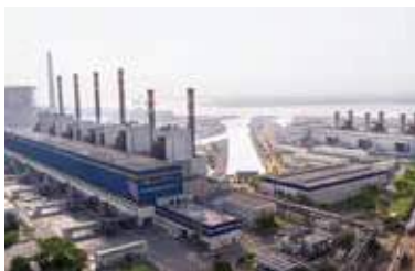
Bin Qasim Power Station I (840MW Thermal Power Station). 4 x Hitachi steam turbine. Each of the units can be fired on Gas and HFO.
